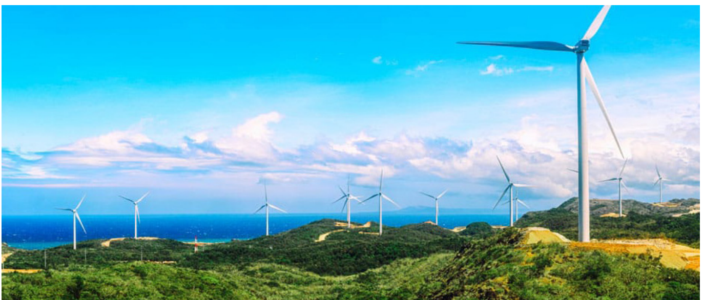
150MW Burgos Wind Project in Burgos, Ilocos Norte, Philippines.
