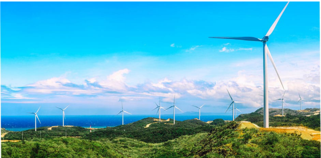
150MW Burgos Wind Project in Burgos, Ilocos Norte, Philippines.
