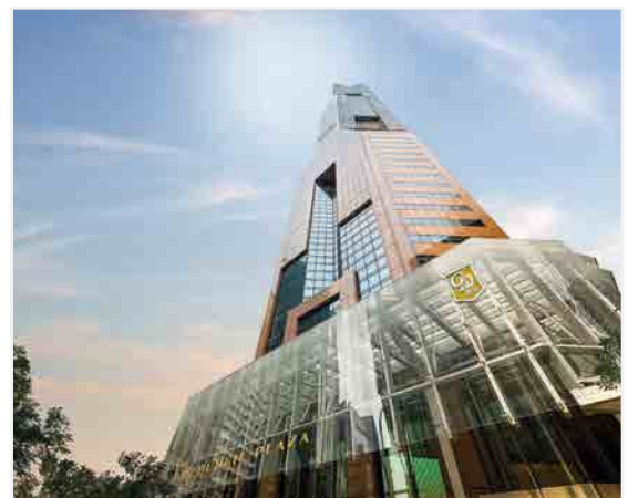
Since its completion in 1996, Republic Plaza – CDL's flagship office building – has maintained its Green Mark Platinum status via regular tracking and enhancements, including major retrofitting of chiller plants and installation of energy efficient lighting with motion sensors to maintain and improve
