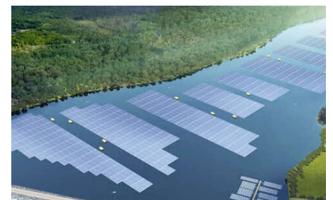
Artist impression of the upcoming 60MWp floating solar system on Tengeh Reservoir – PUB, Singapore's National Water Agency and Sembcorp Industries.
